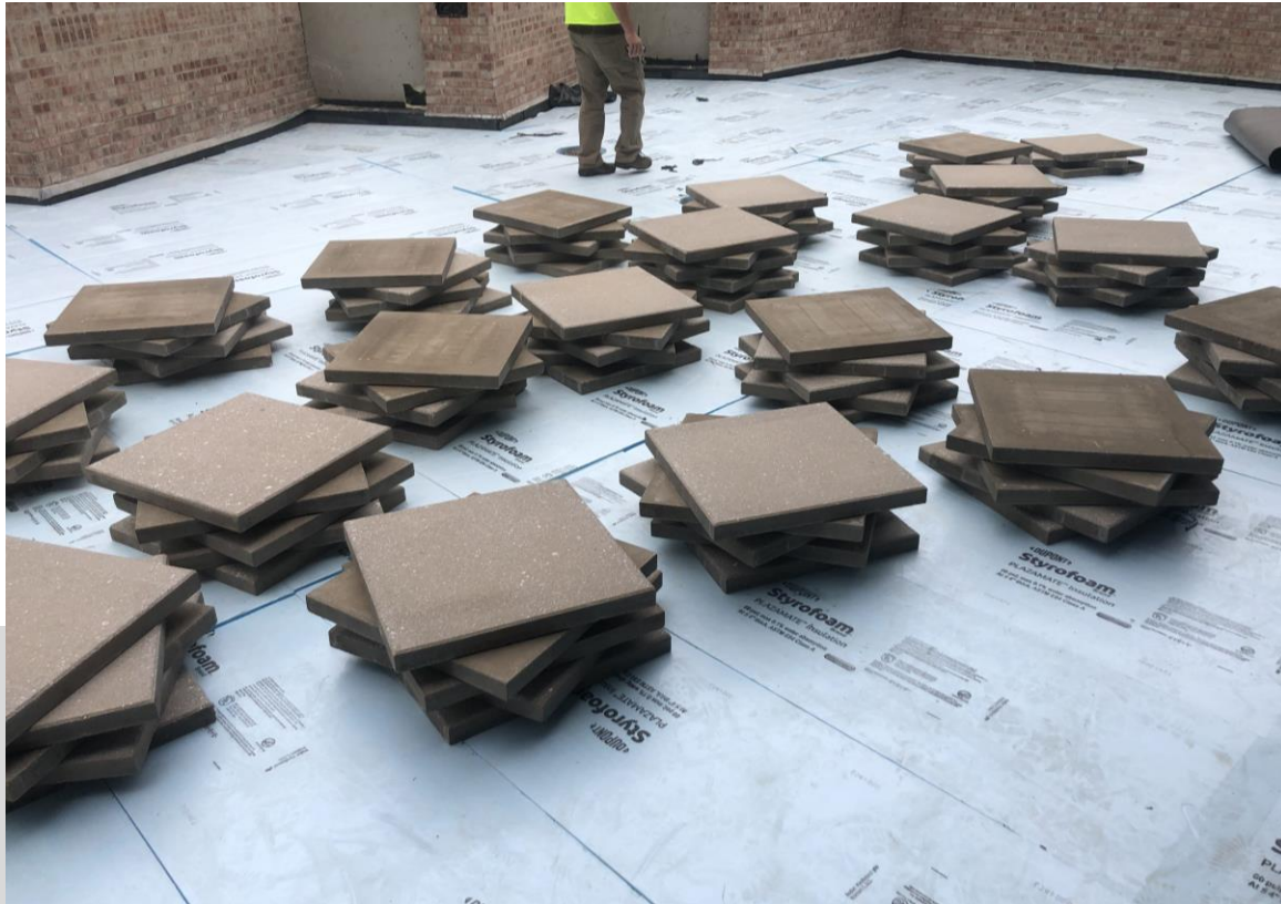
New Addition Patio Pavers Staged for Installation
