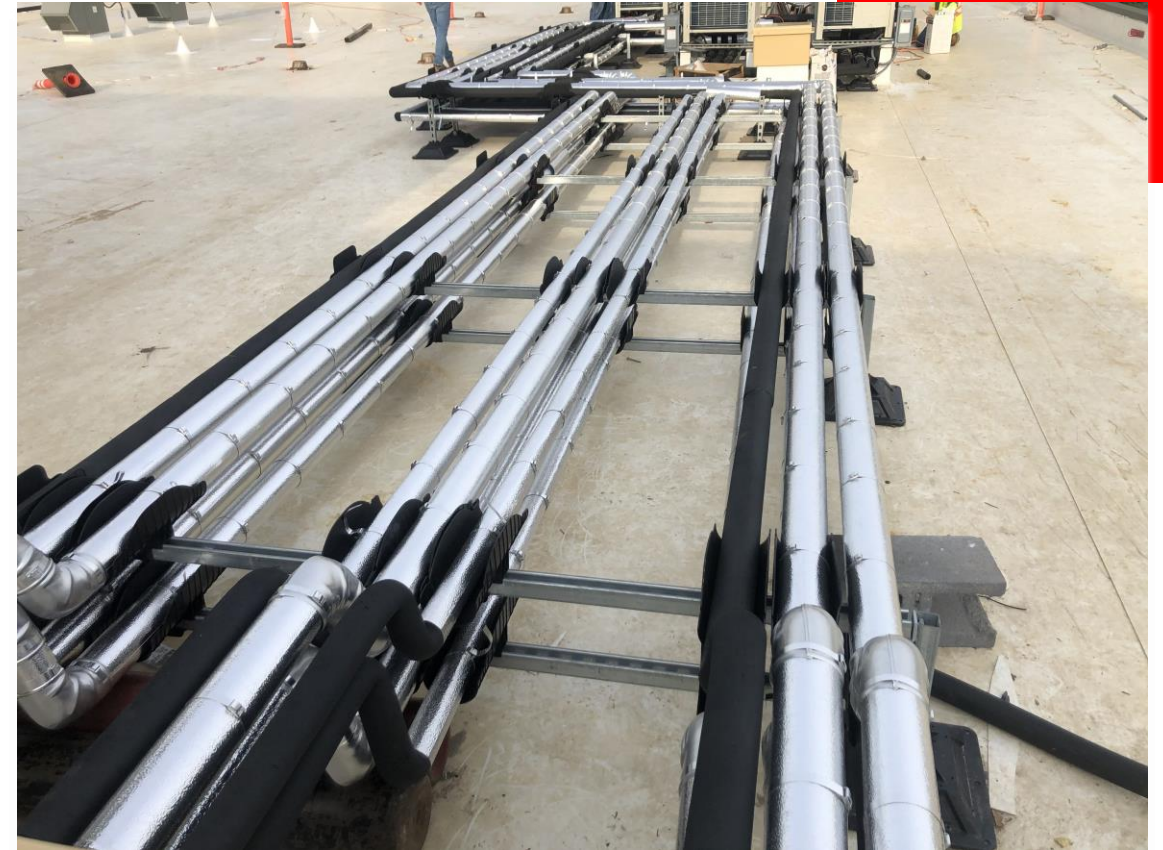
Metal Jacket Insulation Progress on Rooftop Refrigerant Piping
